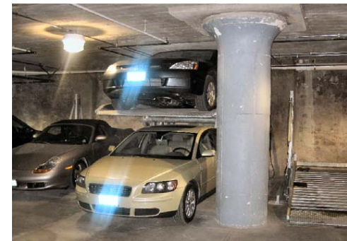
Parking stackers in the basement increase spaces & reduces the need for exterior parking lots
