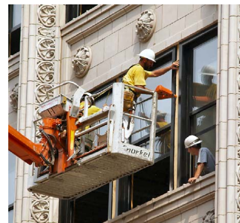
Removing lead paint from windows is an important part of remediation
