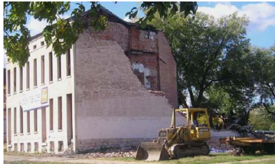
1215 N. Market prior to restoration. The rear wall of the 3 buildings had collapsed taking a portion of the sidewalk as well
